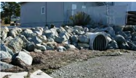
Bay View Padilla Bay Culvert Extension
