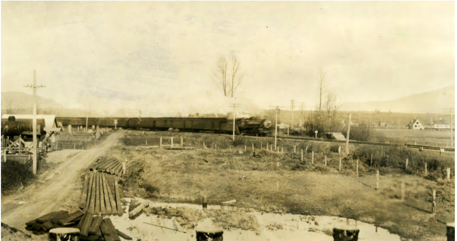
1930s Looking North before Construction
