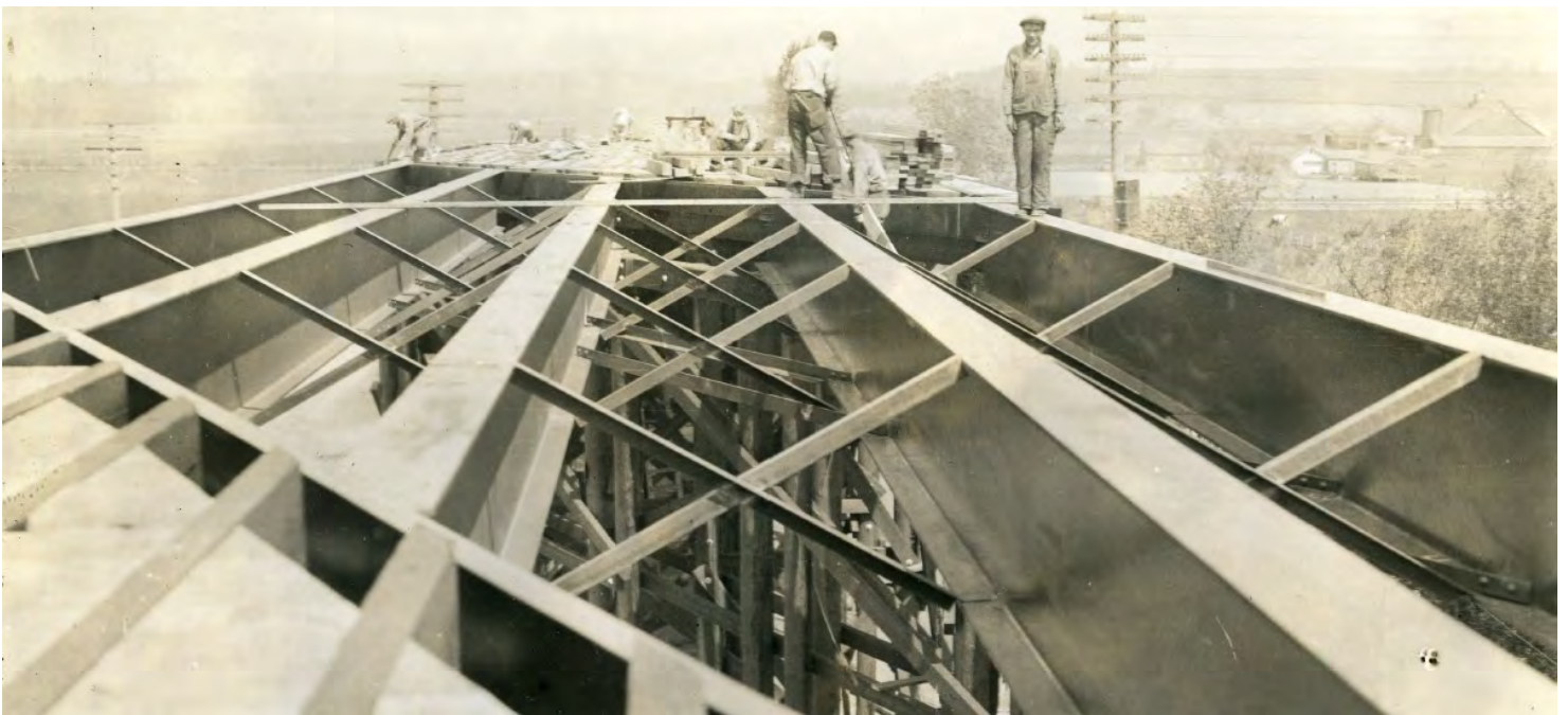
1930s During Construction
