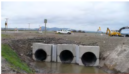
No Name Slough Bypass Culverts
