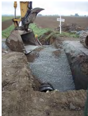
Maupin Road Conveyance Improvement Dike & Drainage District 22 (2008)
