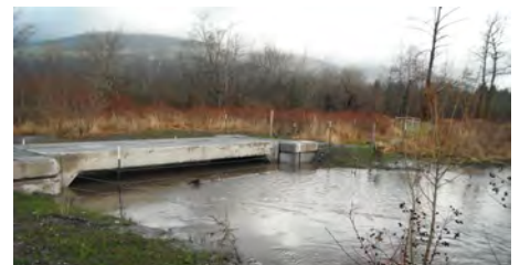
Red Creek Culvert Replacement
