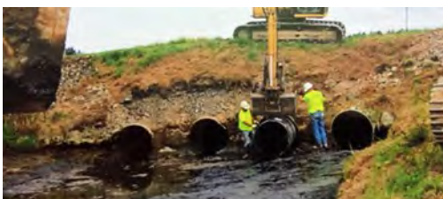
Samish Flood Return Pipe Lining
