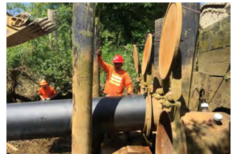
Chilberg Pump Discharge Pipe Lining
