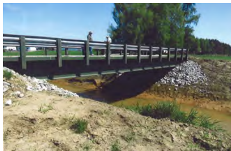
Joe Leary Slough Bridges
